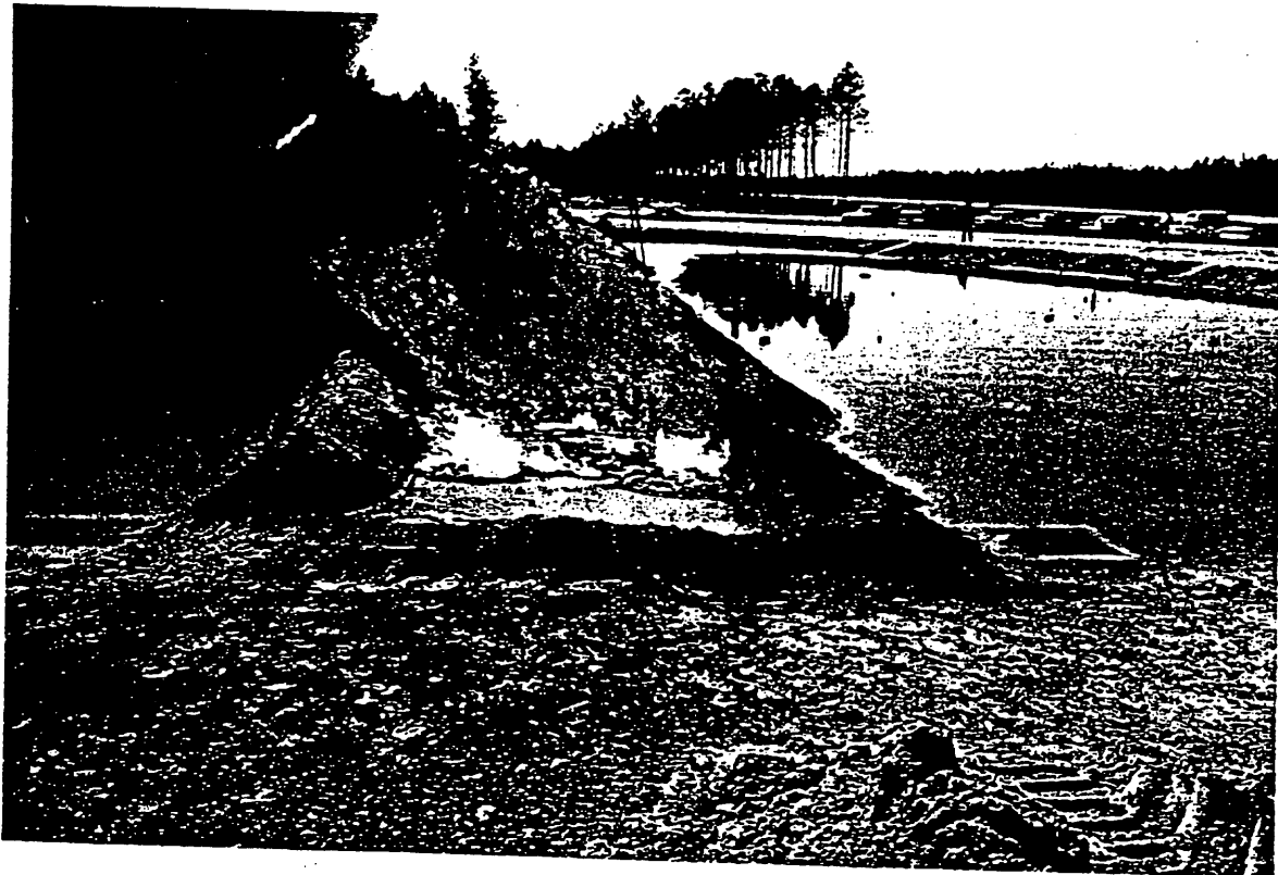
Figure A-6. Fire trench Showing Burnback
